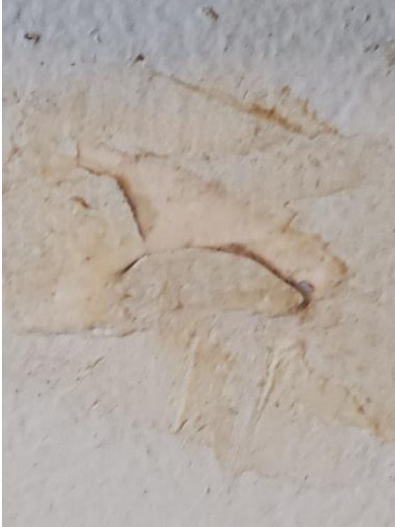
Figure 1 - Patched hole in wall from exploding glass.
