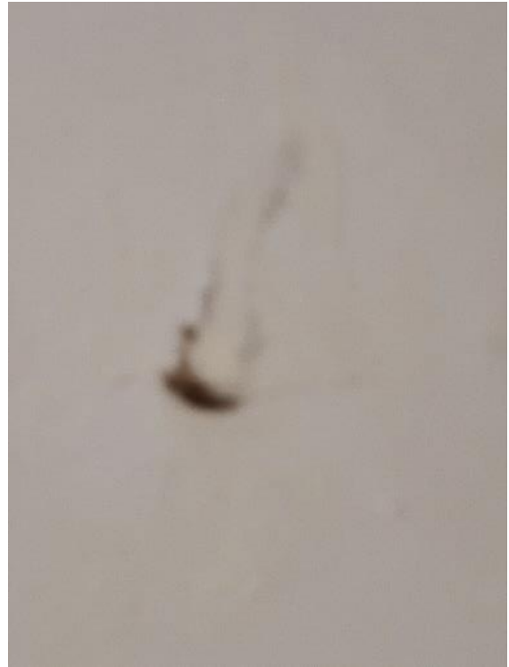
Figure 2 - Patched hole in ceiling from exploding glass (5' away)
